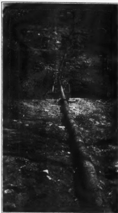
Pipe Line from Pump House to Top of Quarry
